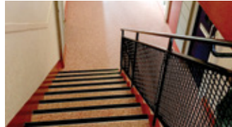
Renovating Communal Areas for Social Housing
