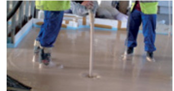
How To Avoid Screed Failure
