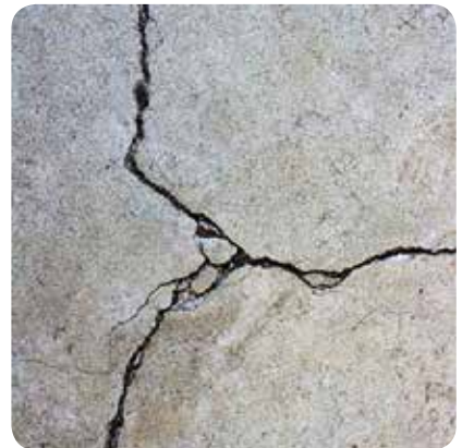
Wide Cracking
