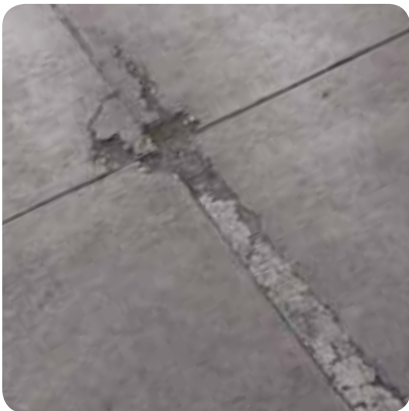
Spalling Joints
