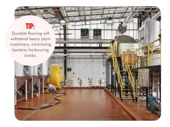
The HACCP International certification program highlights the importance of seamless and impervious flooring, as seams, joints, grout lines and gaps can become breeding sites for bacteria, fungi, mould and mildew. Making sure that the floor provides a seamless surface will help the cleaning regime quickly wash any unwanted substances out of the area.
