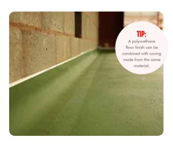
install an expansion joint between the floor and coving. Both products are also independently rebated into the concrete.
